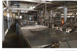
Sami Labs' Customized Extraction Line Sami Labs has also invested in a custom extraction line for its Bangalore, India, facility. This state-of-the-art extraction line is designed to produce high-potency botanicals and other natural products. The facility is ISO 22000 certified, HACCP compliant, and has a clean environment.
